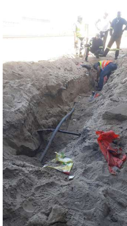
Figure 3: Cable fault repair.
